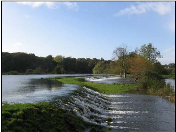
Overtopping at Postwick Marshes
